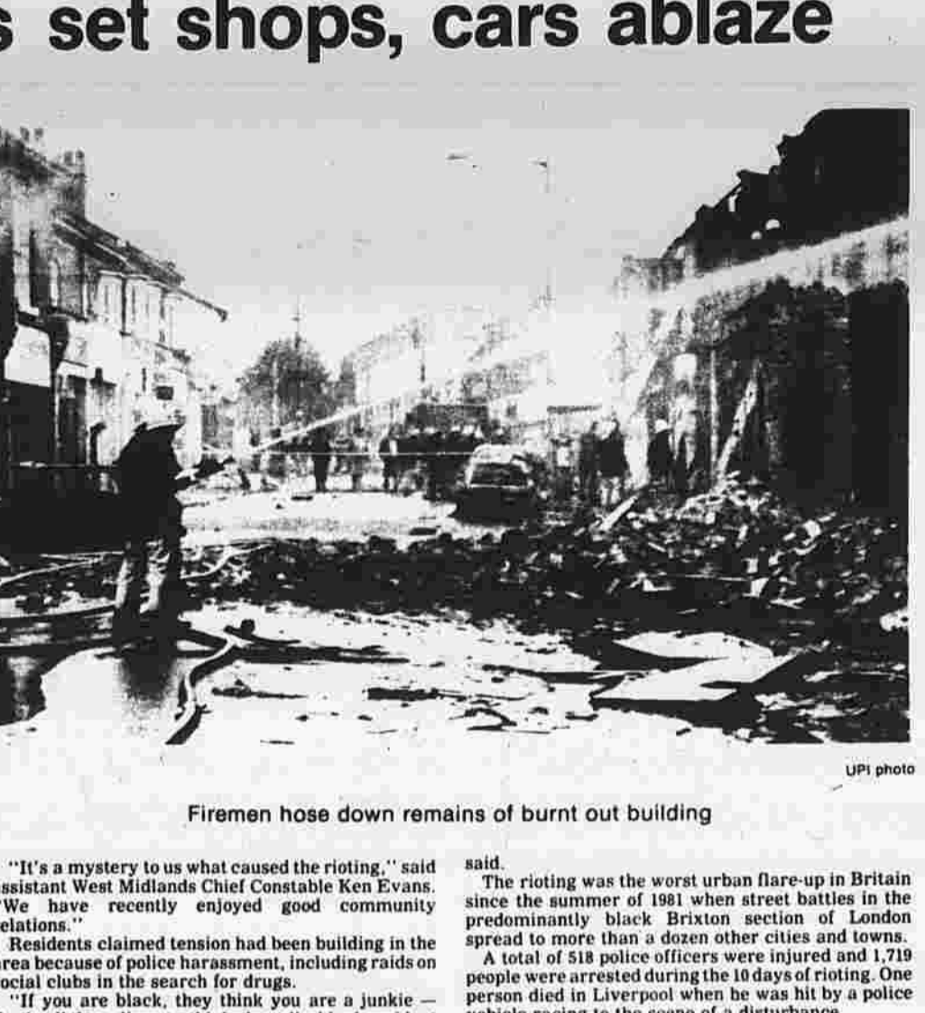
Firemen hose down remains of burnt out building
